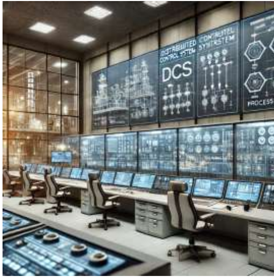
Gambar 4. 5. Distributed Control Sistem (DCS)
