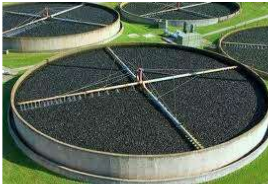
Gambar 7.8. Trickling filter (Sumber: (Cahyana, 2013))
